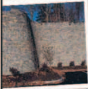
Municipal Parking Lot, Town of Wilton, Maine, in VERSA-LOK Weathered Mosaic
