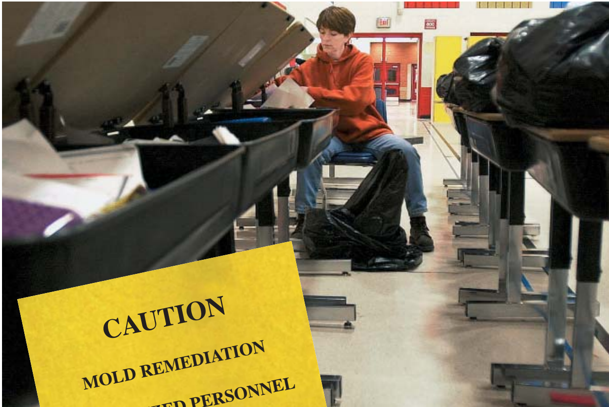
A custodian at Chavez Elementary School empties students' desks for mold remediation three months after the school opened.
