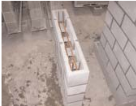
Figure 2 - Bond beam reinforcement.
